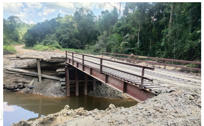
Sg. Linei Puteh I-beam bridge
